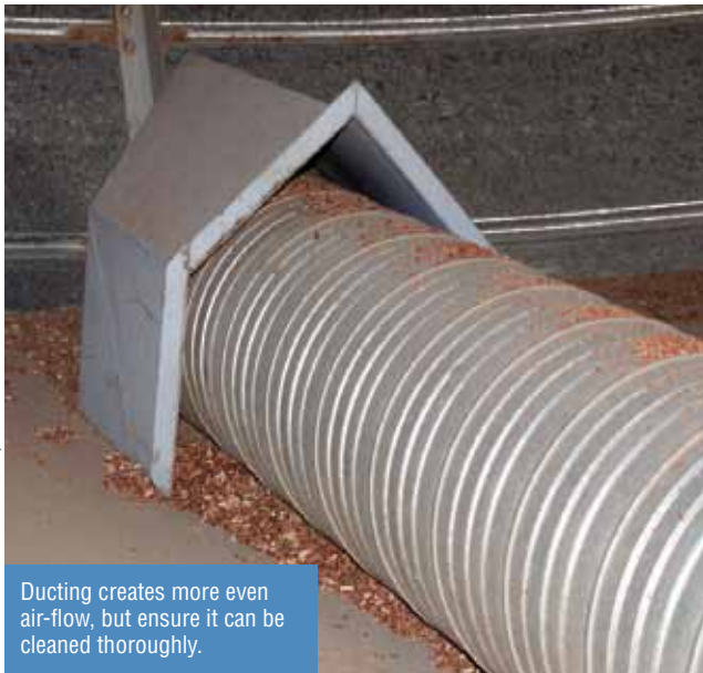
FIGURE 1 AIR MOVEMENT WITHIN AN AERATED SILO
