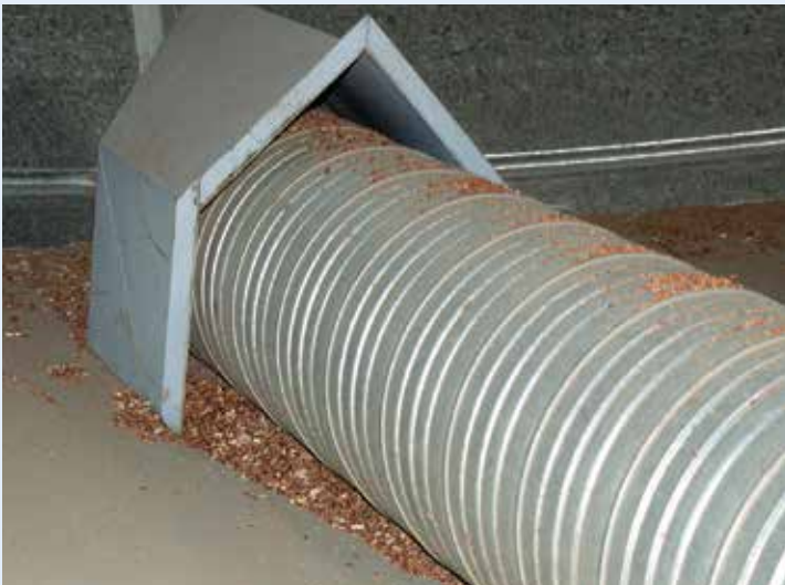
Easy cleaning: Ducting creates more even air-flow, but ensure it can be cleaned thoroughly.
