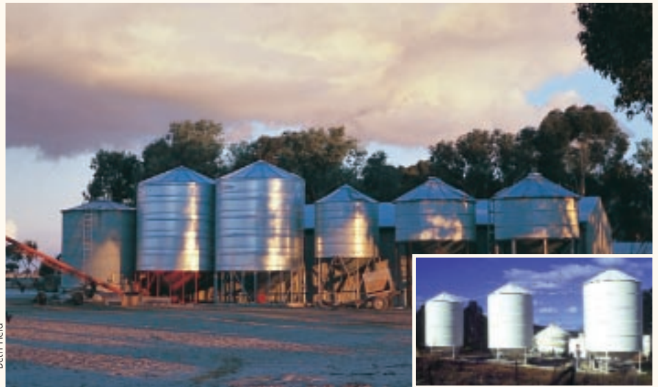
Effective storage can enhance grain quality. Inset: For on-farm grain storage, CSIRO recommends raised, sealed silos, painted white and sited on a concrete base to enable a residue-free environment.
