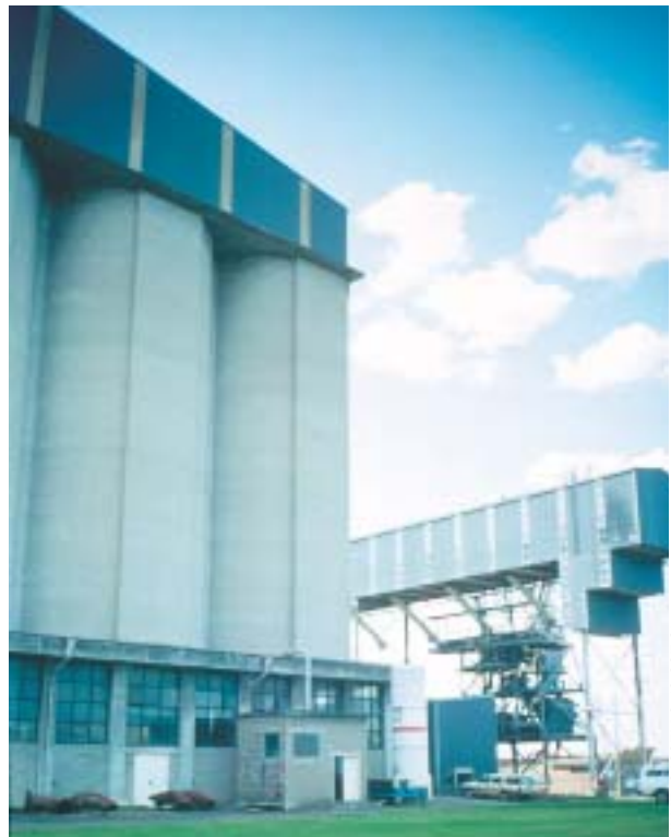
Bins at Newcastle (NSW) export terminal under nitrogen disinfestation treatment before export. The nitrogen storage is at the base of the bins.
