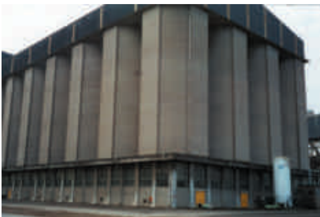
Figure 1. The Newcastle nitrogen treatment plant showing the 20 t tank that serves the closest 16 large bins.
