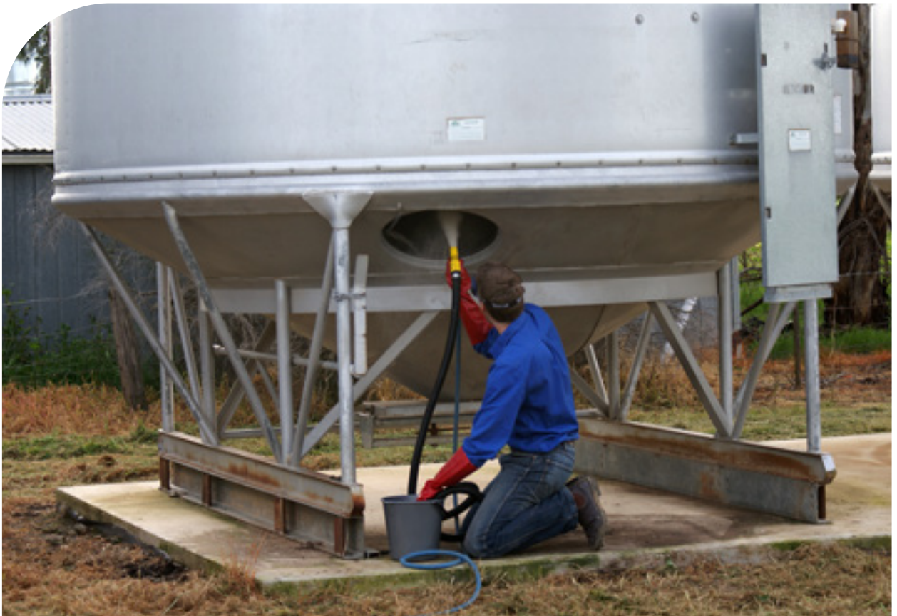
Applying a Diatomaceous Earth (DE) treatment to internal storage surfaces controls any remaining storage pest insects following the physical clean-up (Source: GRDC)
