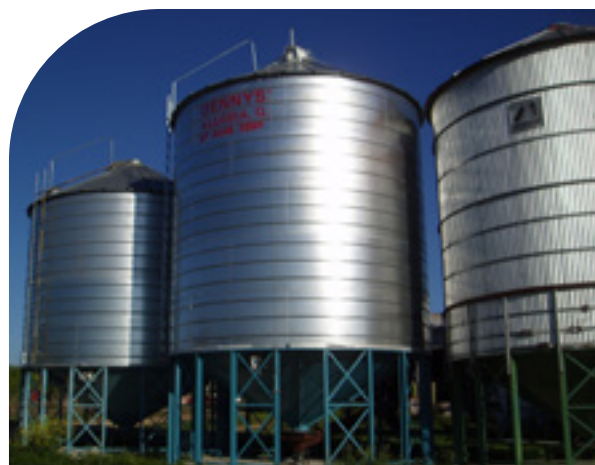
Typical cone-based aerated, sealable silos that are suitable for pulse storage
