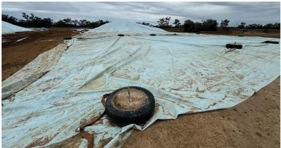
Bunkers are used without side walls to minimise the time requirement for covering and securing bunker tarps at harvest.
