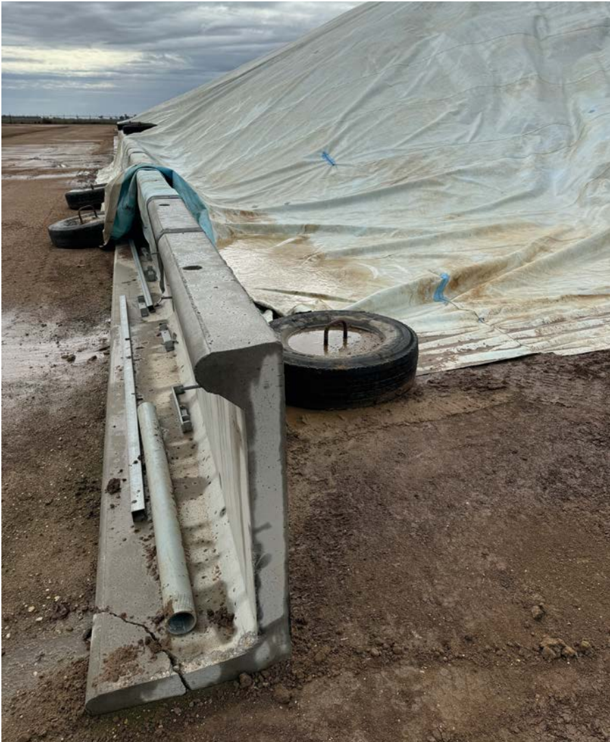
Bunker walls can increase capacity without increasing bunker footprints but require management when unloading.
