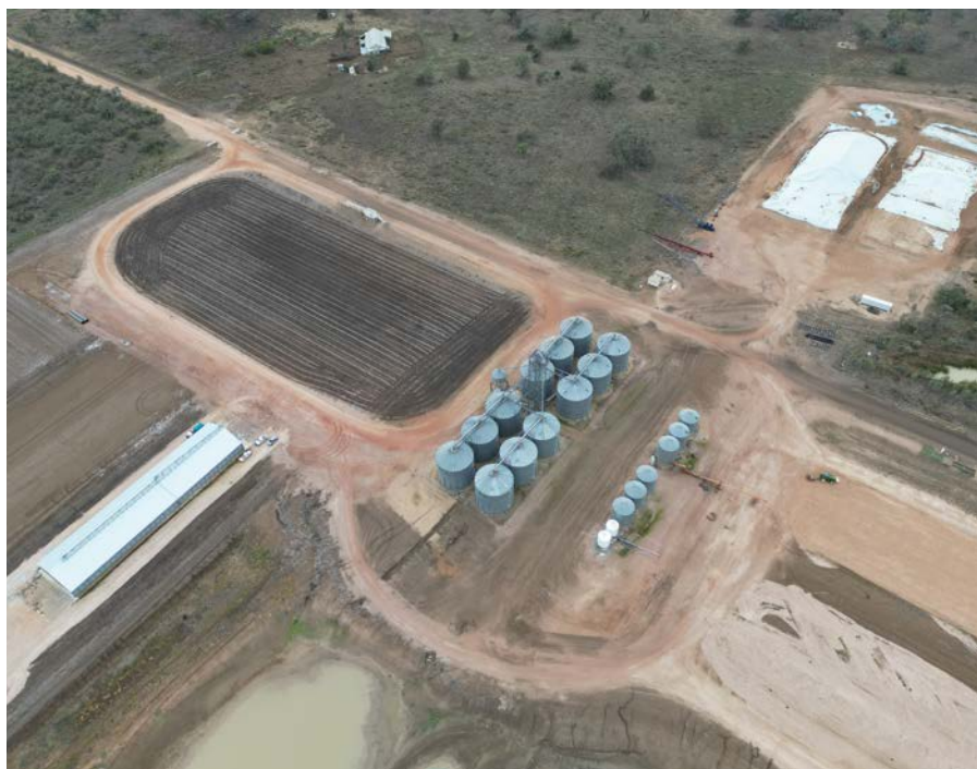
South Bunarba incorporates a range of storage options including sheds, bunkers and upright storage.
