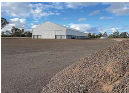
Extensive hard stand at either end of the shed.
