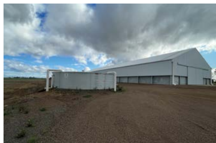
The shed feeds two 175,000L water tanks with rainwater.
