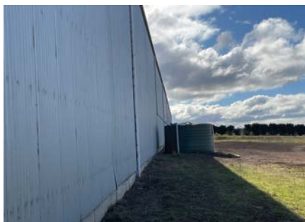
Rainwater is captured in a series of 22,500L poly tanks.
