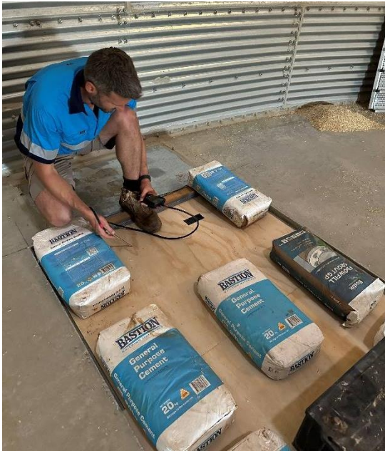
Figure 10: In-situ testing performance of the axial flow fan using the aeration trench covered with ply-board to create a tunnel to measure airflow.
