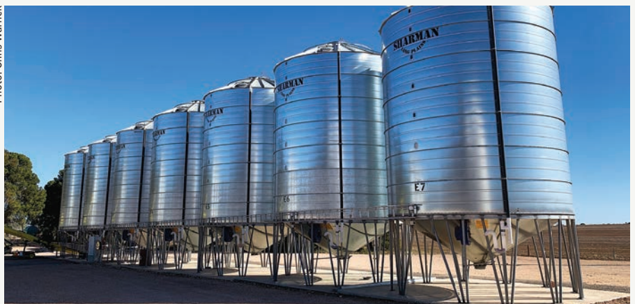
Sulfuryl fluoride should be used in rotation with phosphine to prevent the development of resistance. Gas-tight sealable storage is required to control all life stages of grain storage pests.
