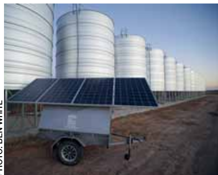
A power source trailer was custom-designed and positioned to maximise solar capture.
