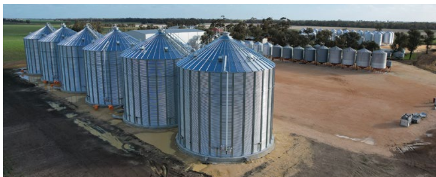
Photo 3: The choice between flat- and cone-bottom silos should consider unloading efficiency, grain segregation, optimum silo size, loading and unloading logistics, and cost. (Source: Chris Warrick, Primary Business)
