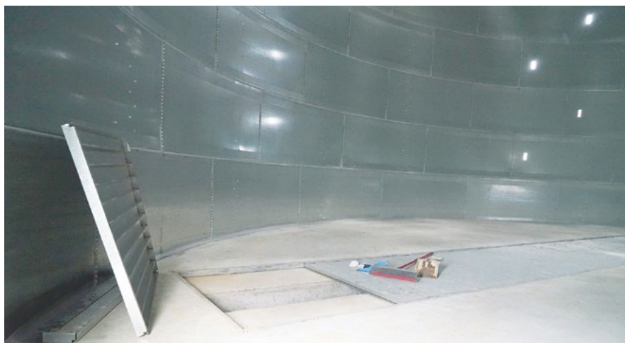
Photo 7: In-floor aeration ducting in flat-bottom silos, which can be removed for cleaning, is ideal. (Source: Chris Warrick, Primary Business)
