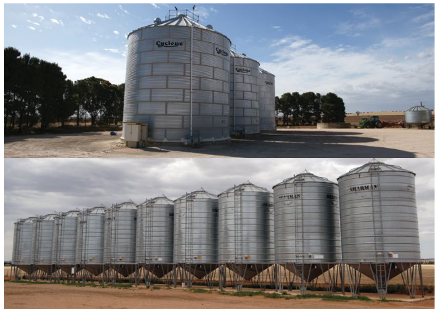
Photo 2: Flat-bottom silos (photo top) and cone-bottom silos (photo bottom) remain the most popular on-farm grain storage options. (Source: Chris Warrick, Primary Business)
