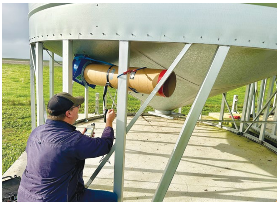
Photo 9: Ensure manufacturer quoted airflows have been field tested. Research has identified variation between theoretical and actual fan performance. (Source: Chris Warrick, Primary Business)
