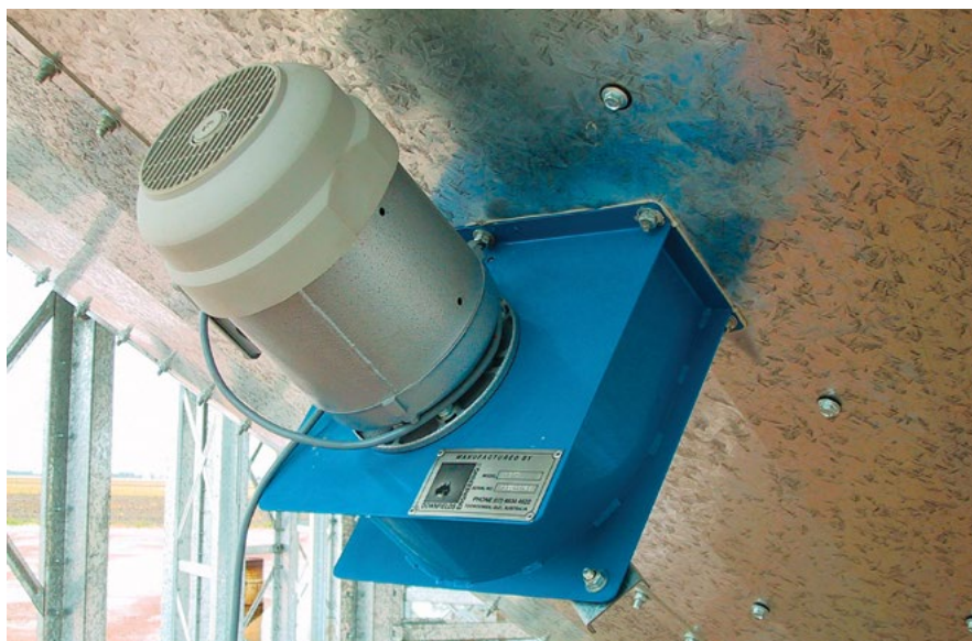
Photo 1: If over-moist grain can't be dried immediately, hold it under aeration cooling until drying equipment is available. (Source: Phillip Burrill, DAF QLD)
