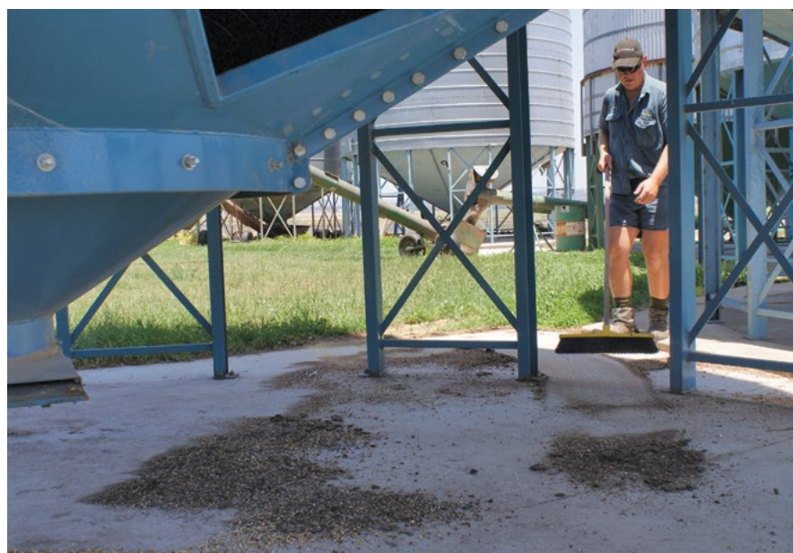
Photo 2: A concrete slab under silos makes cleaning easier. (Source: Chris Warrick, Primary Business)
