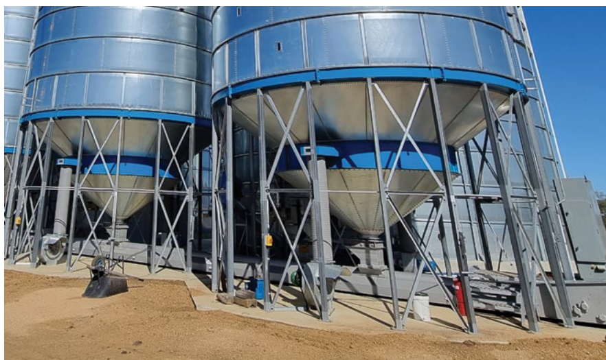
Photo 2: A purpose-built silo for aeration drying has a large fan capable of more than 15 L/s/t with ducting right around the silo cone. (Source: Alex Conway)
