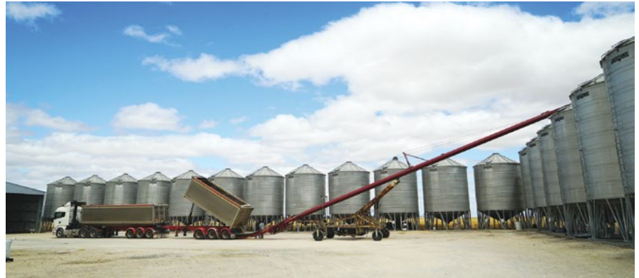
Photo 2: Having a large gravelled area around silos enables machinery to be moved into position safely. Always fill silos from the centre to avoid uneven loading. (Source: Chris Warrick, Primary Business)
