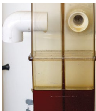
Photo 3: Ensure the pressure relief valve is filled with sufficient oil to be level with the middle indicator mark. (Source: Chris Warrick, Primary Business)
