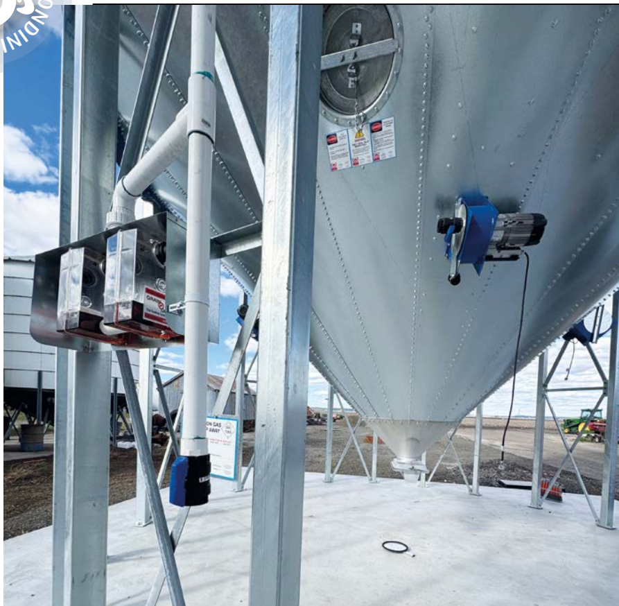
Fit for purpose: Gas-tight sealable silos should meet the Australian Standard AS 2628:2010.
